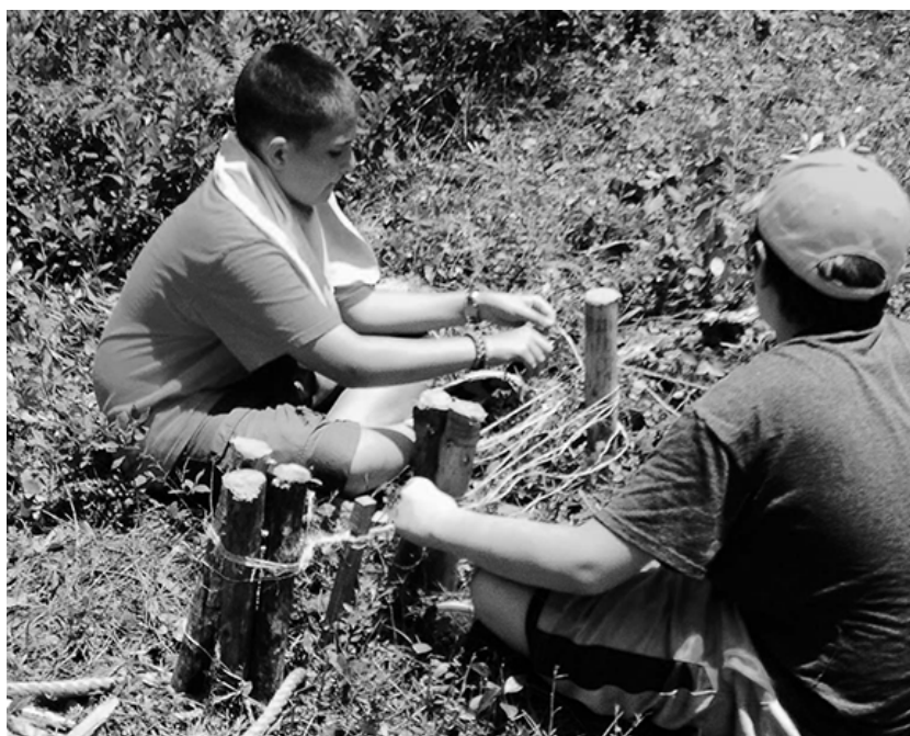
A Scout uses binder twine to connect the two-stake set to the single stake for their monkey bridge.
